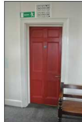
Existing door adjacent to new opening
