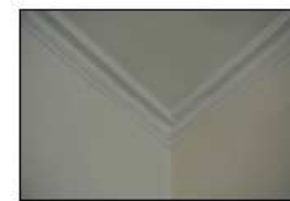
Existing plaster cornice
