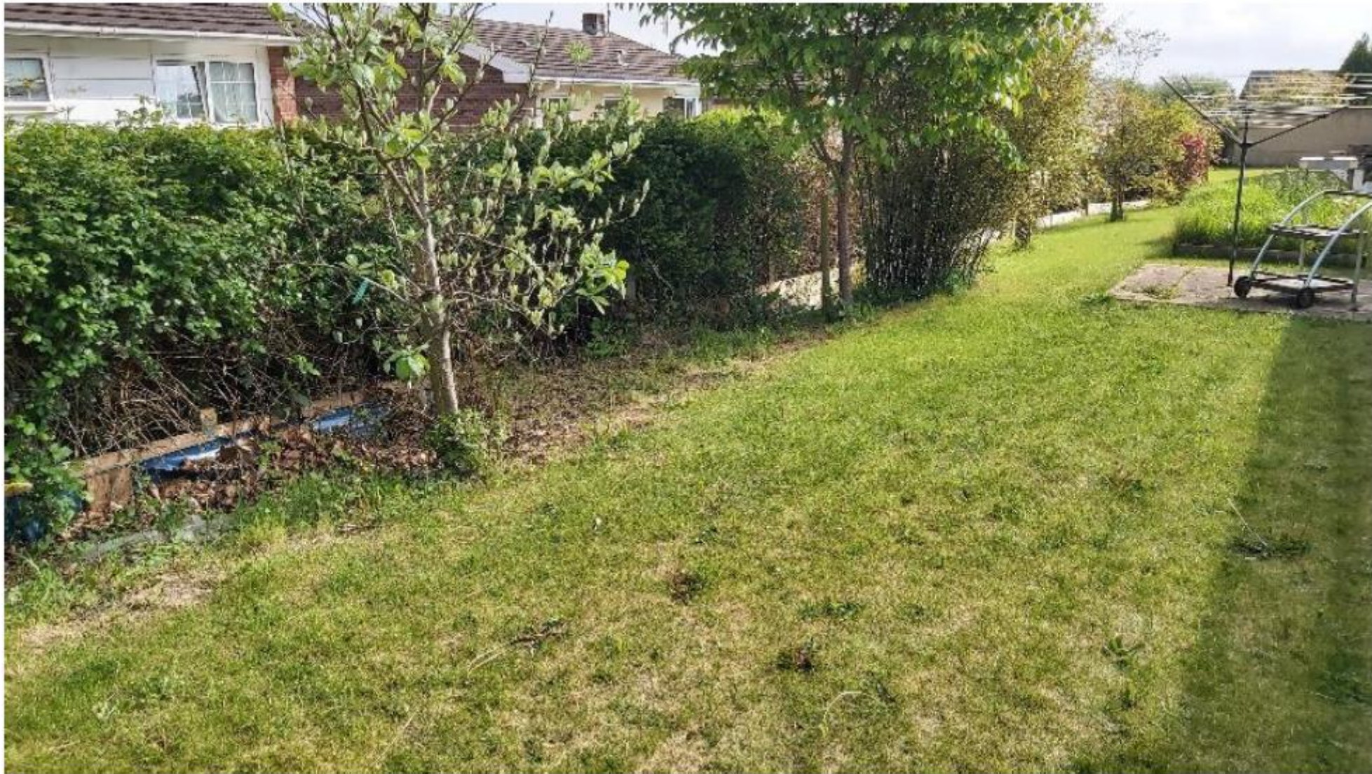
Photo from structural report undertaken prior to installation of gabion wall showing ground level.
